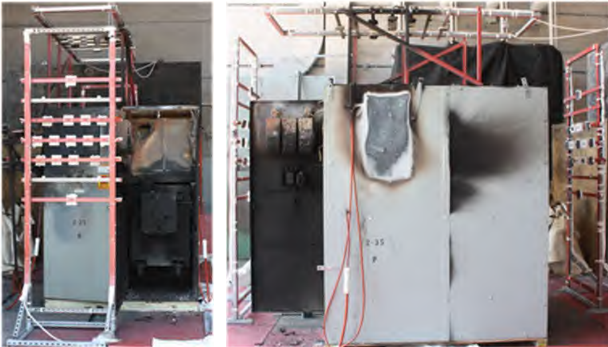
Fig. 49. Enclosure Post-Experiment 2-35 (Left – front view with Rack #1 in front of Enclosure “O”, Right – side of Enclosure “P”).
