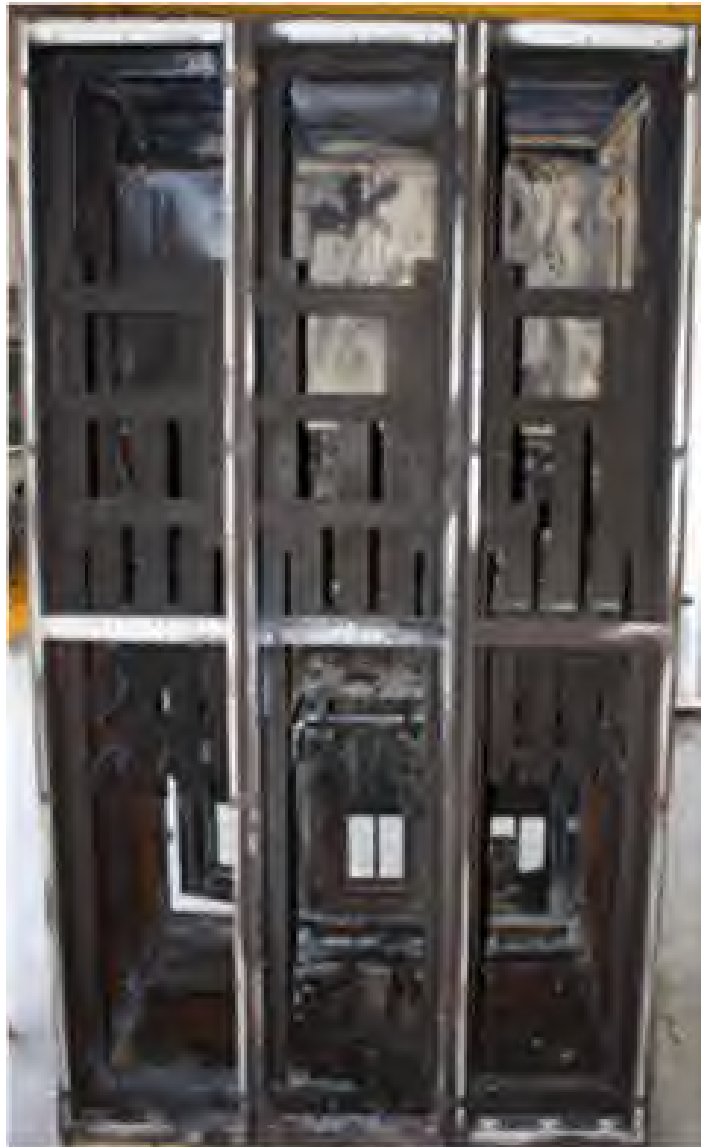
Fig. 168. Post-Experiment internal view from rear.
