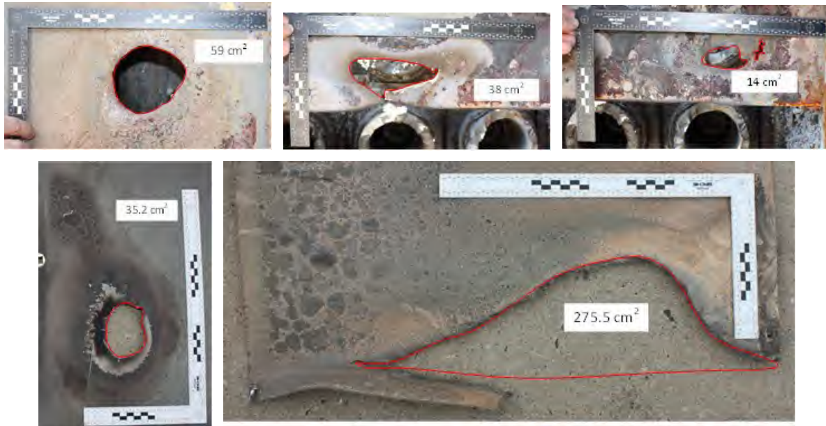
Fig. 198. Post-Experiment 2-39 Enclosure “M” Breaches. Top – internal panels near secondary run-backs, Bottom – internal bottom bus panels.
