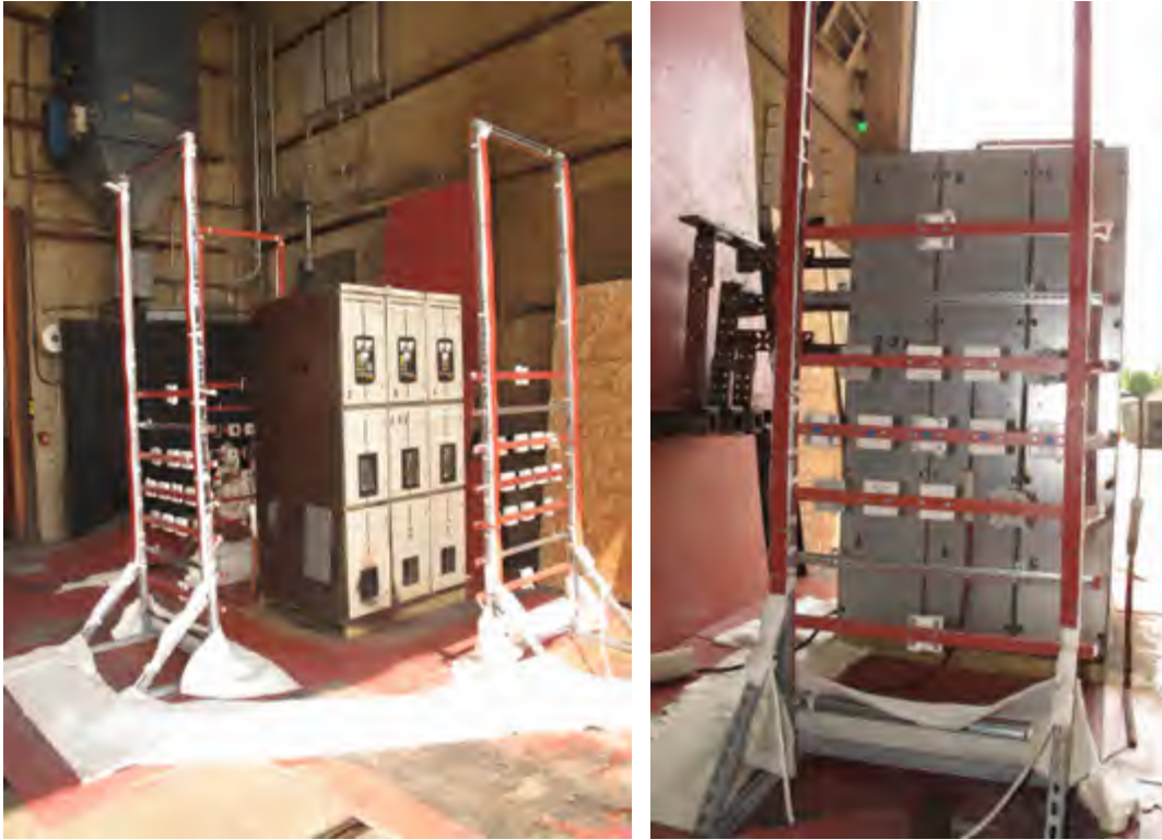
Fig. 166. Pre-Experiment 2-33B in test cell. Left – front corner view, Right – experimental device viewed from rear.
